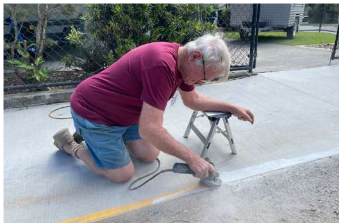
Dave removing the Yellow Line for a Loading Bay
